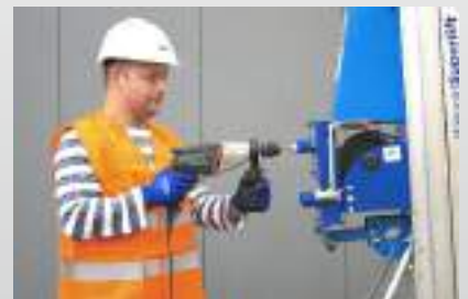
drive with drilling machine
