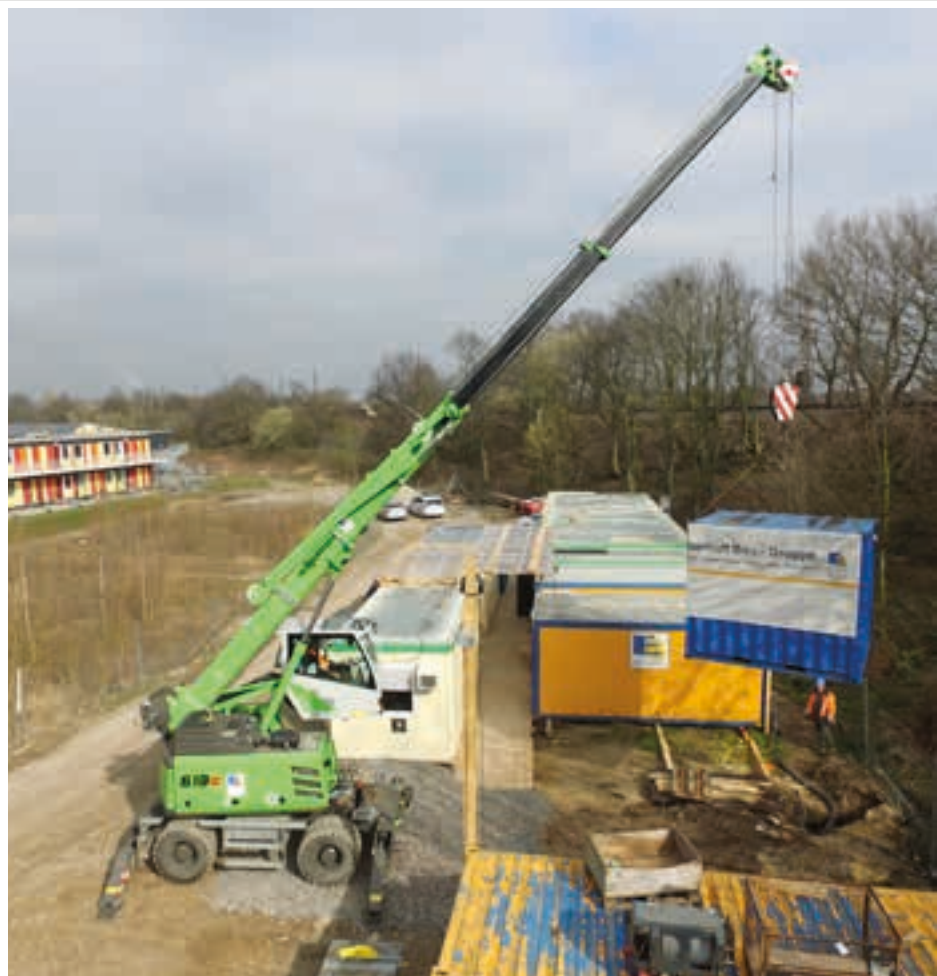
The 613 E Mobile being used for lifting activities and logistics tasks at a railway construction site
