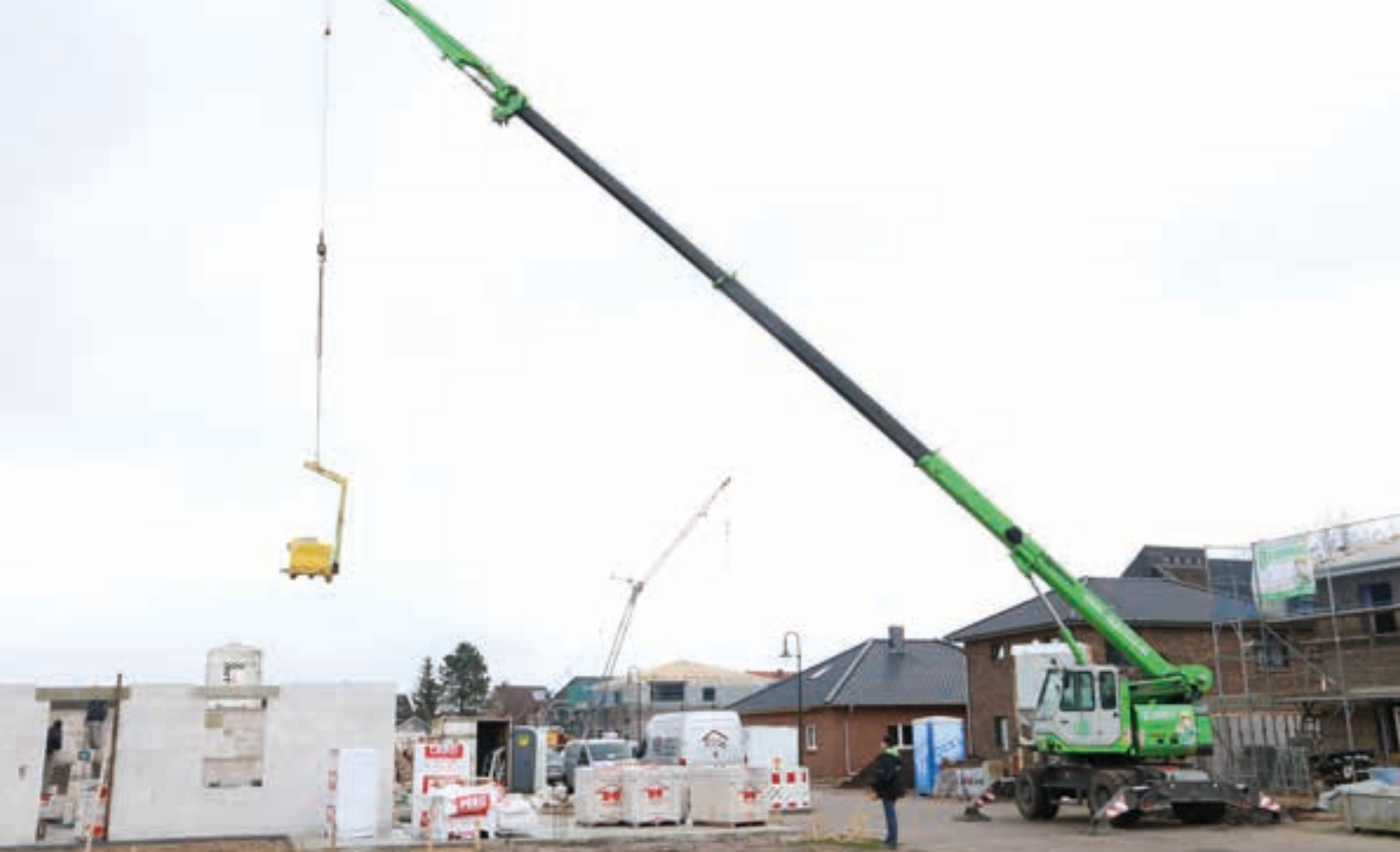
The 613 E Mobile optimizes construction site logistics during the process of completing a detached house in Germany.
