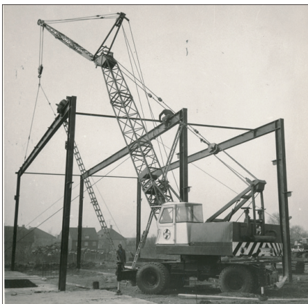
1972: rope-driven SK 15 with plastic operator cab
